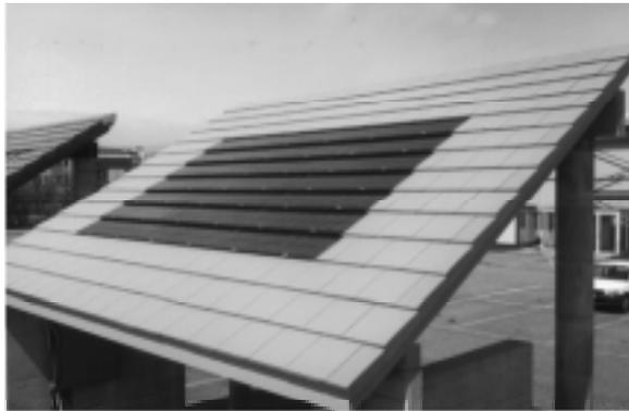
Fig. 2. The roofing system from Braas: an interesting combination of standard concrete based tiles and glass-glass customized modules.
