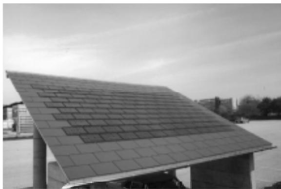
Fig. 1. : The new roofing system Sunslates (by Atlantis) displayed at the Demosite.
