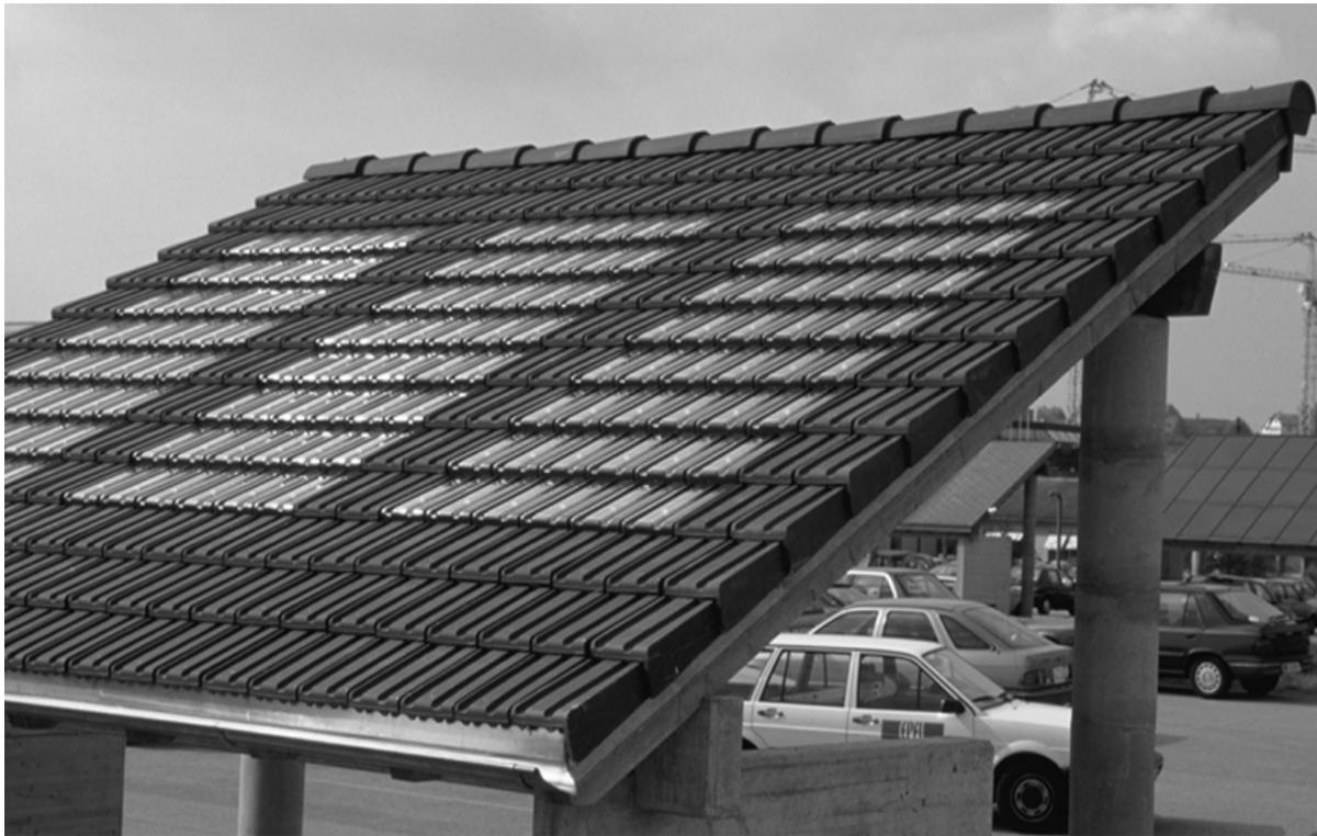
Fig. 2. : The new roofing tile Star Unity: three fields of PV tiles surrounded by ceramic standard tiles. Thanks to a well thought out connection system, the mounting time is very close to that of conventional tiles.
